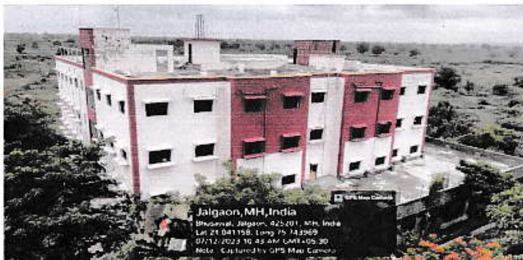
COLLEGE BUILDING FRONT VIEW
